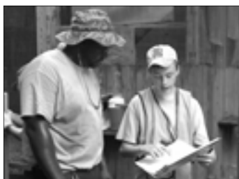
Charlie Queen directs other scouts and volunteers in the construction of new doors
